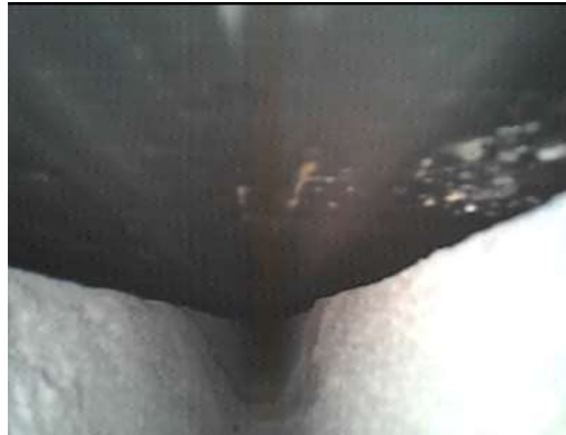
Full scale mockup Inspections
