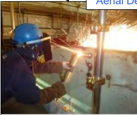
Demonstration of Heat Cutting
