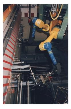
Remote controlled dismantling with Top-Tec Bagger – Kahl NPP
