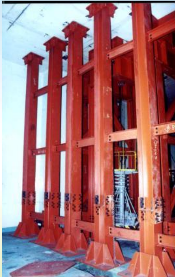
Floor column support below transfer rout
