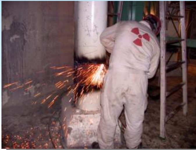
Remove original vessel support
