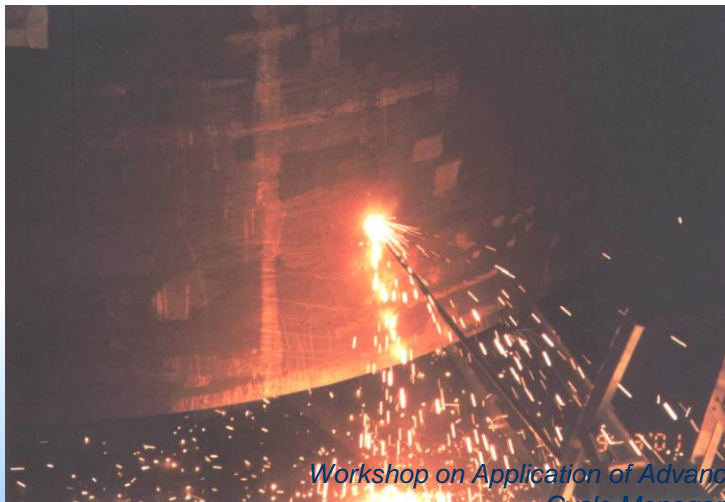
Greifswald Oxygen lance cutting
