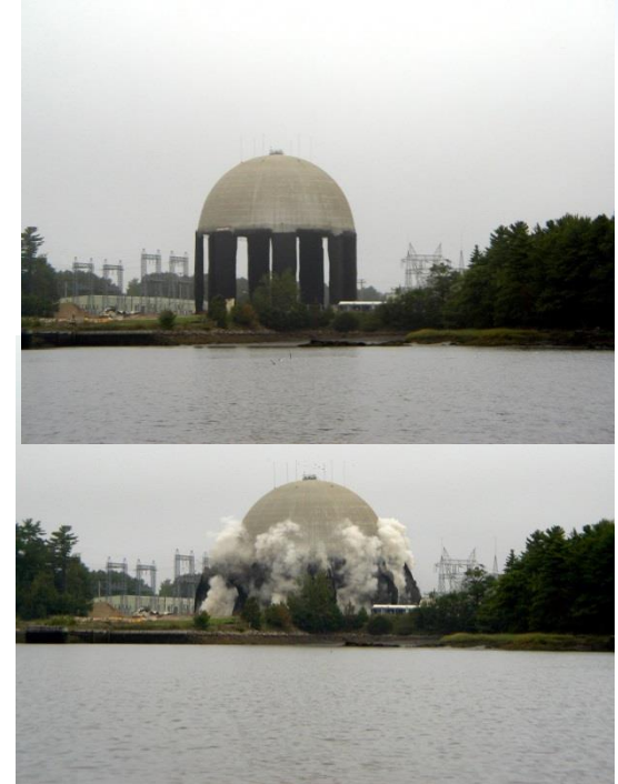
Maine Yankee concrete containment demolition
