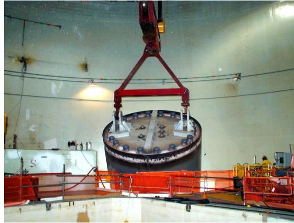
Maine Yankee vessel lifting
