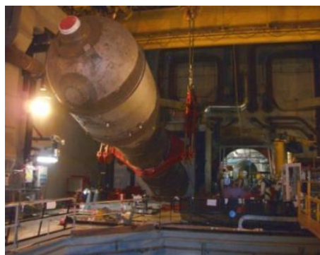
Bugey pumping station dismantling
