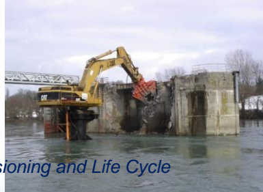
Bugey pumping station dismantling
